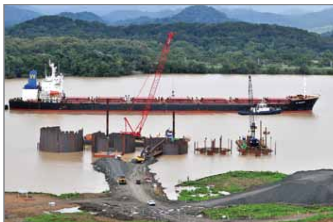
Ongoing work on the Borinquen cofferdam.
