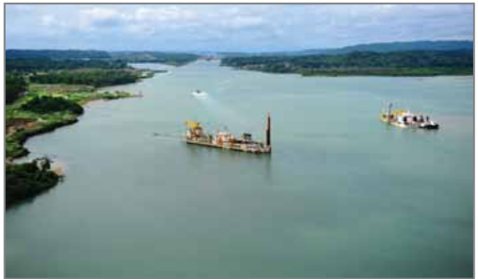
Equipment deployed for dredging activities on the Atlantic side.
