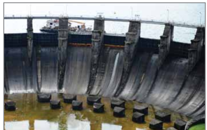
Extension of Gatun Spillway gates
