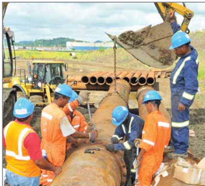
Installation of dredging pipe in the PAC-4 disposal site.
